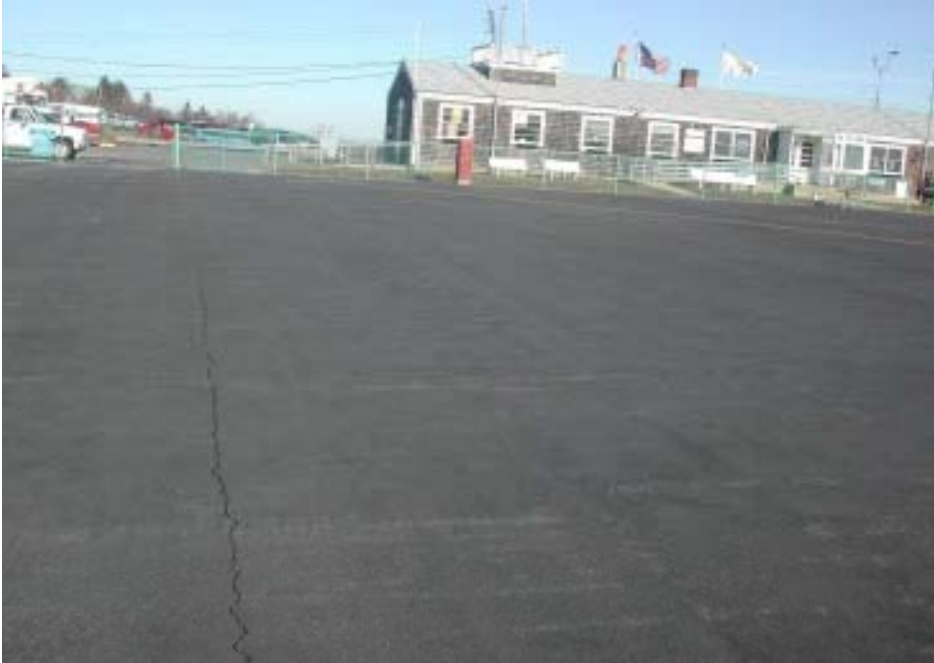
Figure A2-37 Terminal Apron with Low to Moderate Severity Cracking
